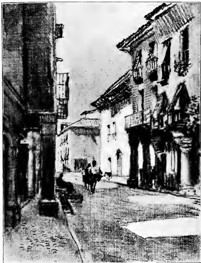
CALLE MAJOR, ALCALÁ
